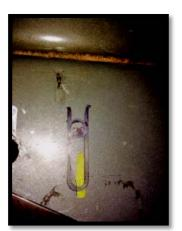
**Step 6:** Remove clip. Use a ½" drill bit and drill out the center mark. Slide the 3/8 clip back into position so the threaded part is aligned with the hole.
