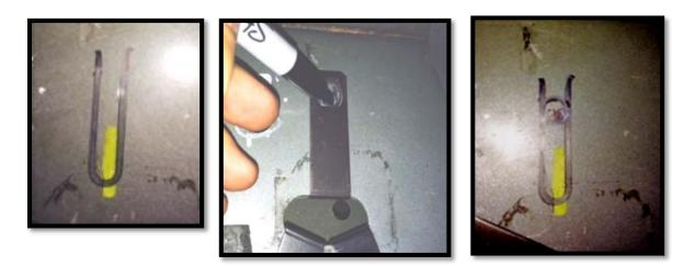
**<u>Step 6</u>**: Remove clip. Use a <sup>1</sup>/<sub>2</sub>" drill bit and drill out the center mark. Slide the 3/8 clip back into position so the threaded part is aligned with the hole.
