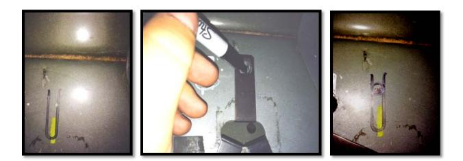
**<u>Step 6</u>**: Remove clip. Use a <sup>1</sup>/<sub>2</sub>" drill bit and drill out the center mark. Slide the 3/8 clip back into position so the threaded part is aligned with the hole.
