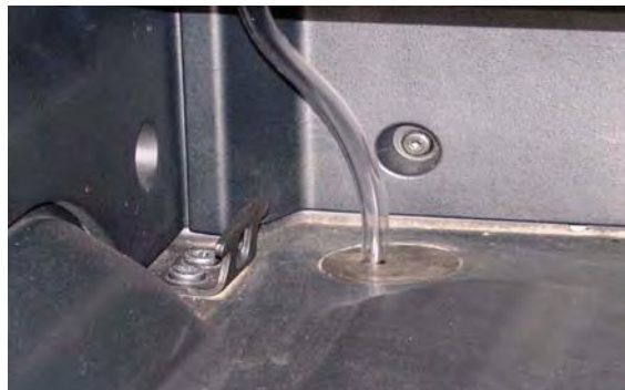
Fig. 15a Drivers' front corner – drain tube installed through plastic bed bolt covers.
