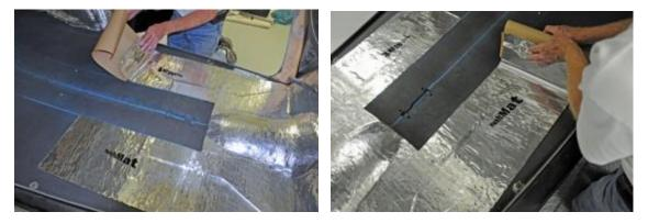
**31.** The sheets were then laid down along these guide lines. This will produce a very straight and neat installation.
