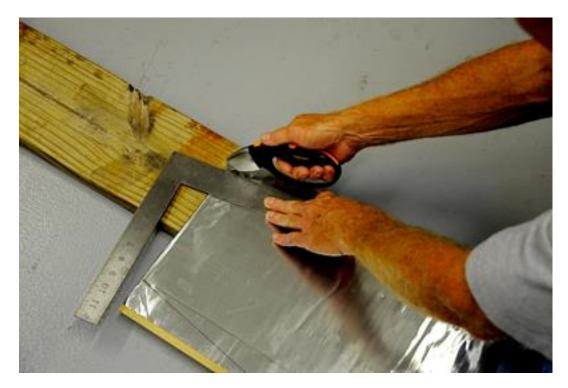
7. The HushMat Ultra can be cut to fit any area using a straight edge and utility knife on a piece of wood as shown here.
