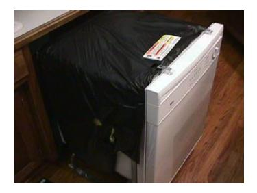
Step 2. Remove the insulation pad from the dishwasher.
