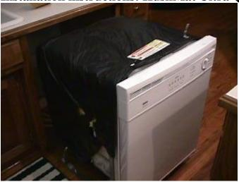
Step 6. Gently push the appliance back into the cabinet, bend the bracket back to the underside of the counter and reinstall the two holding screws. You' are now ready for peace and quiet.
