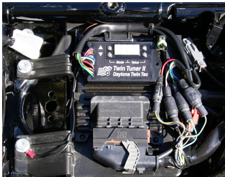
Figure 7 – Completed Twin Tuner II Installation
