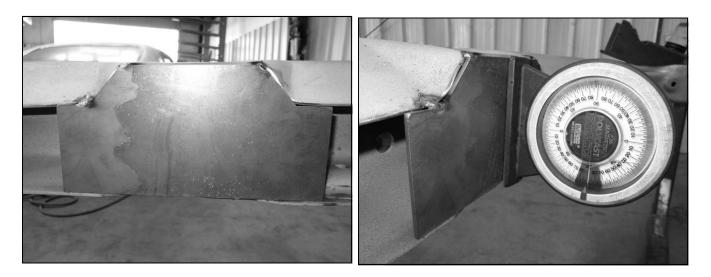
18. Tack backing plate in place as shown with bottom edge of backing plate resting on top of lower rail flange. Make sure that bracket is vertical before proceeding.
