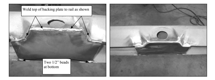
19. Weld backing plate to lower rail flange with two 1/2" long beads at either side. Do NOT add any more weld to bottom of backing plate. Weld top of backing plate as shown to top flange of frame rail. For a cleaner appearance the weld on the top of the backing plate can be ground smooth at this time with a flap disc.
