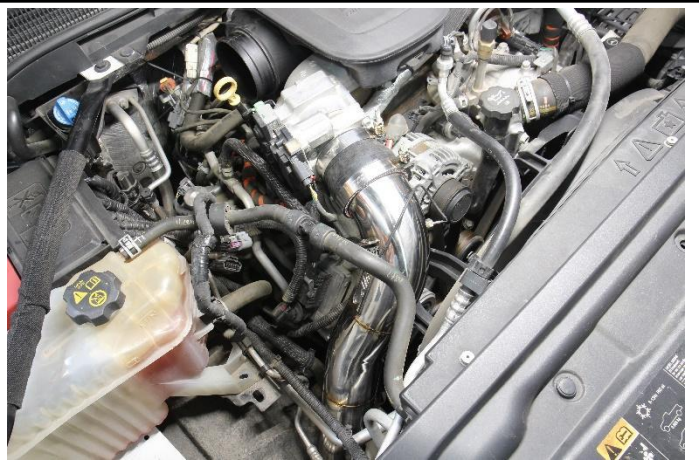
17. Insert the charge pipe into the throttle body coupler. Adjust the charge pipe into position and secure all the t-bolt clamps. Reconnect the air temperature sensor electrical harness.
